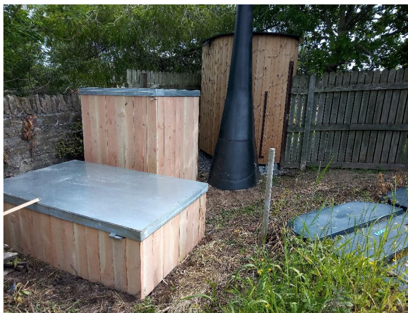
Plate 15. Indicative dry toilet typical configuration.
