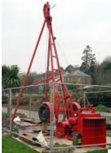
Plate 13. Example of drilling rig to be used for geotechnical investigations on Inis Cealtra.
